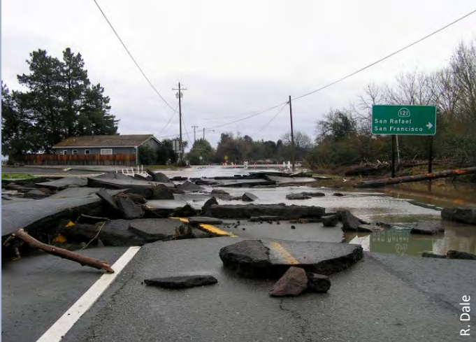
Damage from the December 31, 2005 flood, between Schell and Sonoma Creeks in Schellville, CA at Highways 121 and 12
